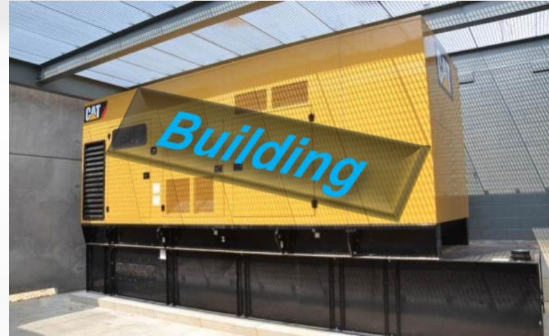
Generator: mounted inside a Permanent Building
